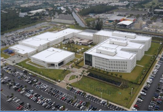
U.S. SOUTHERN COMMAND HEADQUARTERS (SOUTHCOM)
